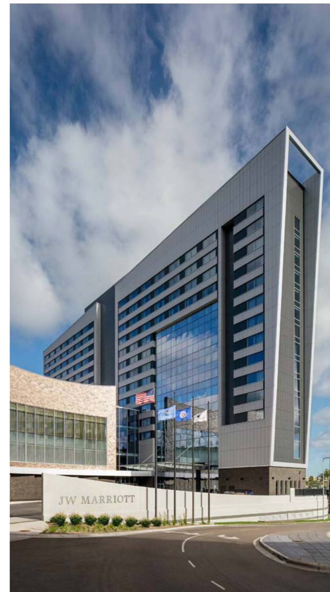
Mall Of America - Architects: Bloomington, MN, USA Photographer: Richard Brine, Minneapolis, USA
