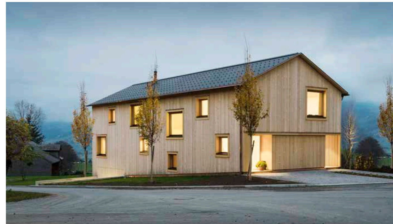
House Rothenbach, Schwarzenberg, Austria. Architect: Baumeister Jürgen Haller GmbH, Mellau, Austria. Photographer: Albrecht Imanuel Schnabel, Rankweil, Austria.
