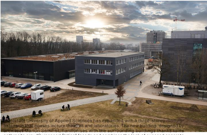
anthracite grey "Swisspearl Patina" façade and combines the look of exposed concrete with the advantages of a lightweight construction. This façade is also robust, offers protection against impact and is low-maintenance. The fibre cement panels are also classified as non-combustible, which increases the safety of the building. With this building project, TH Ingolstadt is focussing on sustainability and modern architecture.
